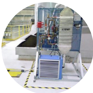
5kW fume condenser prototype at a Urban Waste Power Plant.
